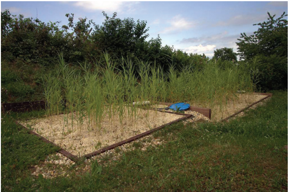
Fig. 2. Constructed wetland for conditioning of drinking water in settlement in NE part of Slovenia.
